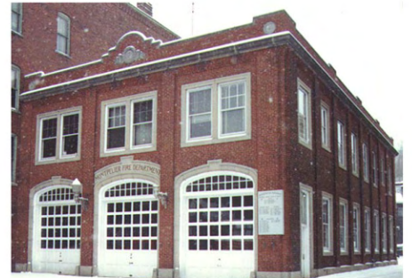
Montpelier voted twice against moving the fire station out of the town center
