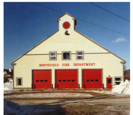
Northfield constructed a new fire station in the town center
