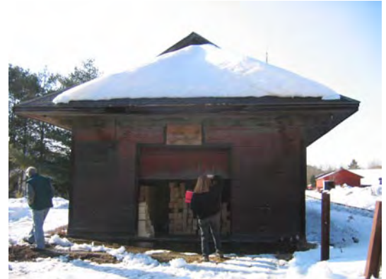
East end where new loading door has been added
