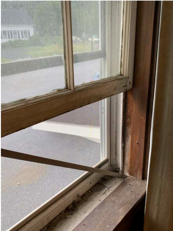
Older windows with storm and screen Are upstairs. Building has little to no Energy efficiencies
