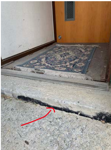
Elevator door open, from outside With detail of concrete step
