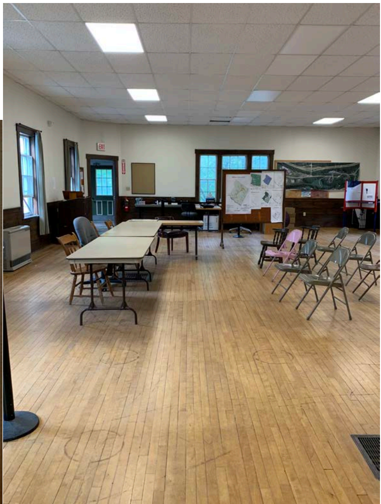
Upstairs common room (voting, committee meetings) Cannot be used for town meeting or community gatherings due to plumbing issues. Currently used by town Clerk during Covid to maintain social distancing
